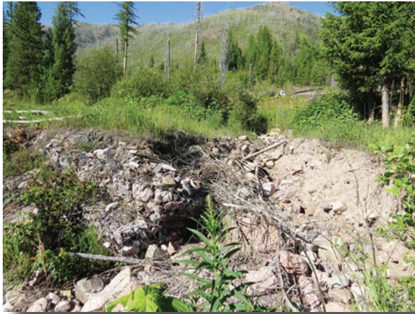
A blown-out culvert in the long-closed Bunker Creek Road 549 in 2014, upstream of bull trout critical habitat.
