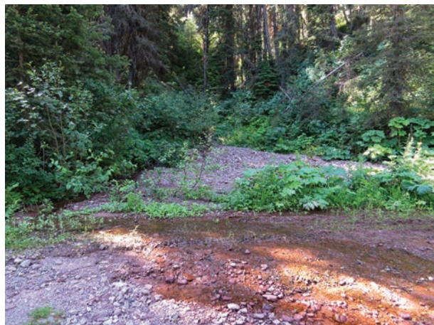
Road 1673 looking upstream at plugged catchment.
