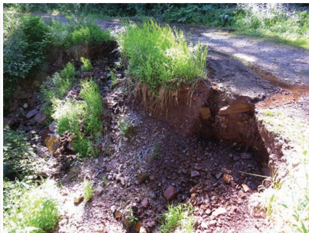
Road 1673 looking downstream at road-fill erosion.
