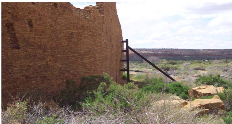
Existing support for three-storey back wall of Pueblo Bonito. (Photo courtesy of Dave Barz)
