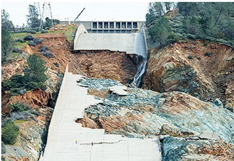
+ The crater in Oroville Dam's spillway has continued to erode as officials have flushed water out of the reservoir at rapid rates. Photo by Florence Low, courtesy of California Department of Water Resources.
