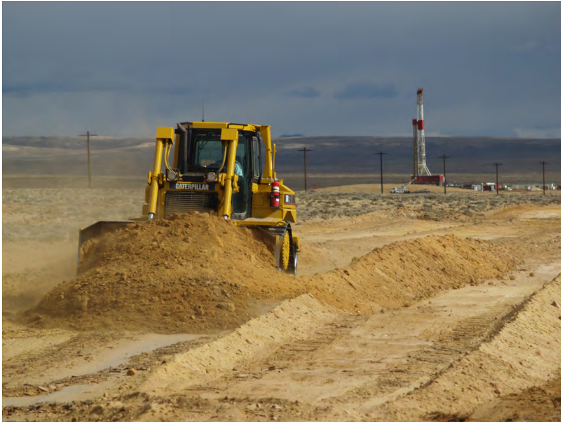
Haul road construction and drilling underway at the Lost Creek project site, October 2012. Erik Molvar photo.
