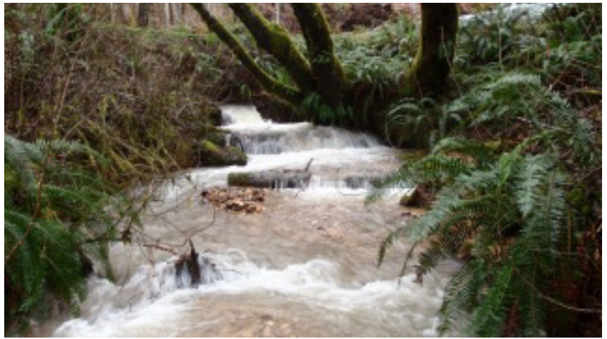
Pre-project, 2010: View upstream of undersized 3-ft culvert hidden in vegetation.
