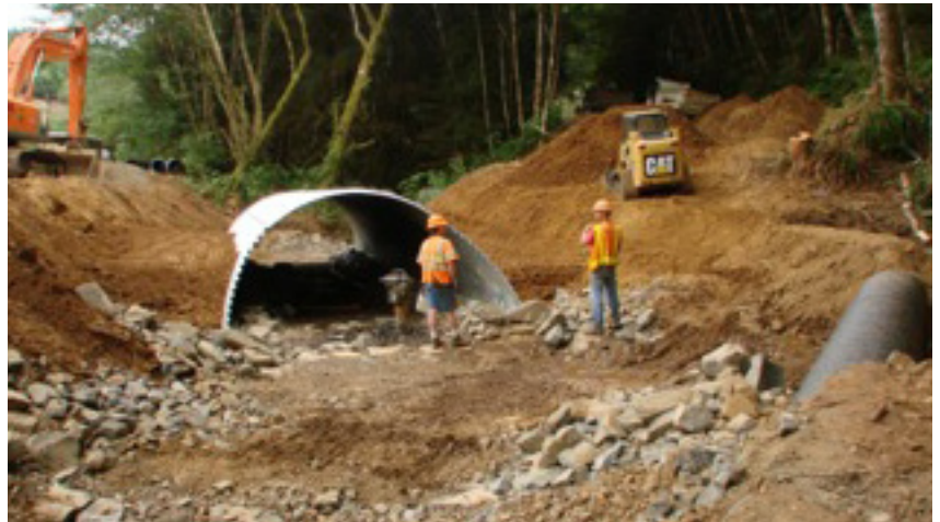
During project, 2011: View downstream with local contractors at work.
