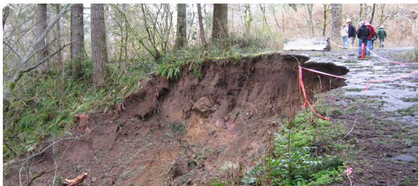
Large road failures can dump truckloads of dirt into creeks—smothering salmon eggs.
