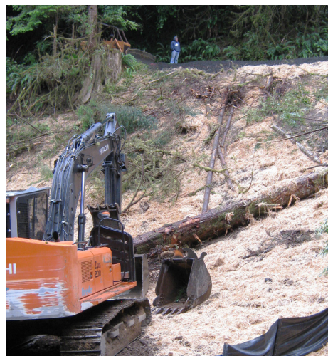
Best management practices include weed-free mulch and screens to keep sediment from entering streams.
