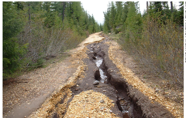
Unmaintained roads funnel sediment straight into mountain streams.
