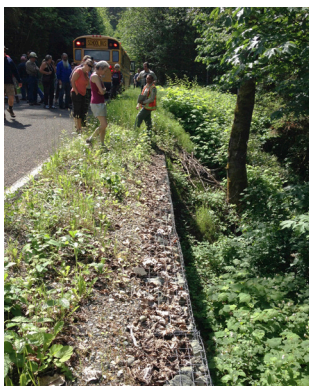
Properly protecting slopes prevents roads from washing out in a storm.
