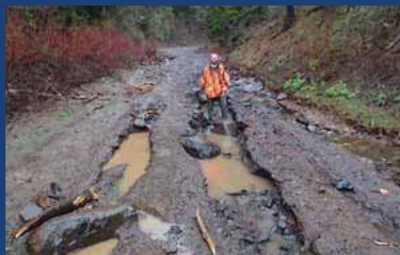
Damage from the April storms. A gullied wheeltrack where flood water was diverted down the road. Photo USDA Forest Service.
