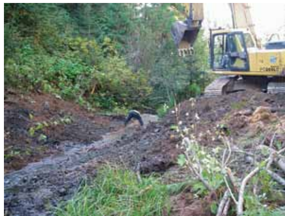
Reconstructing stream channel.
