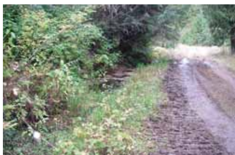
A plugged culvert backs up water along the road. Plugged culverts like this are prone to blow out delivering damaging slugs of sediment to streams.
