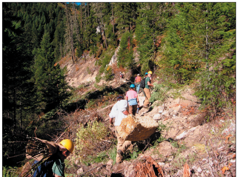
Volunteers doing restoration work. (Wildlands CPR)
