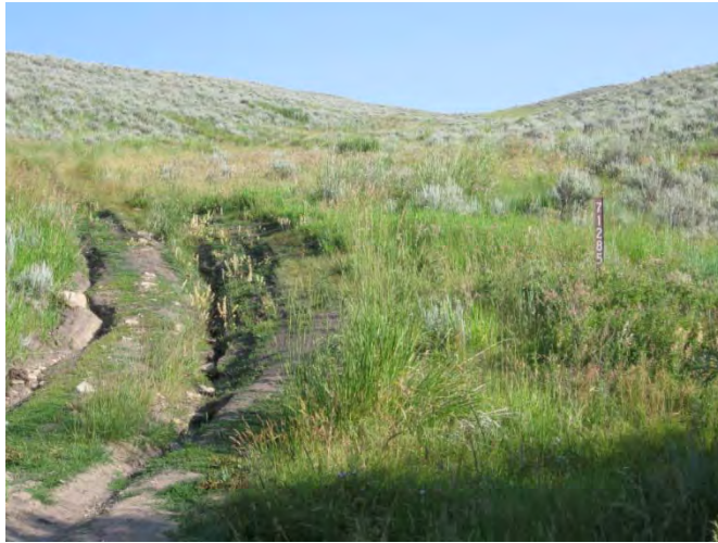
Rd. #21285 in poor condition showing severe gullying
