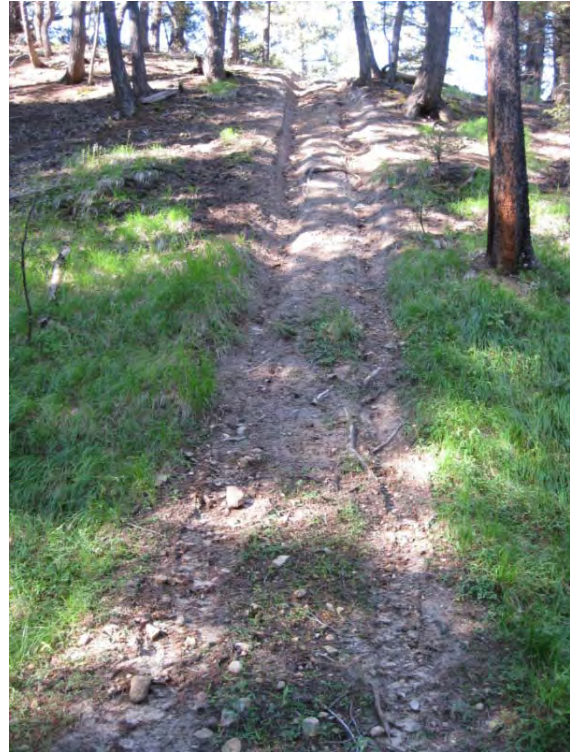
Rutting seen on Tr. #2140 inside the East Pioneer IRA
