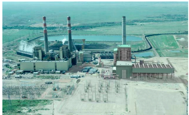
The Comanche power plant with a projected image of the number 3 boiler to the right. Photo by Xcel Energy.
